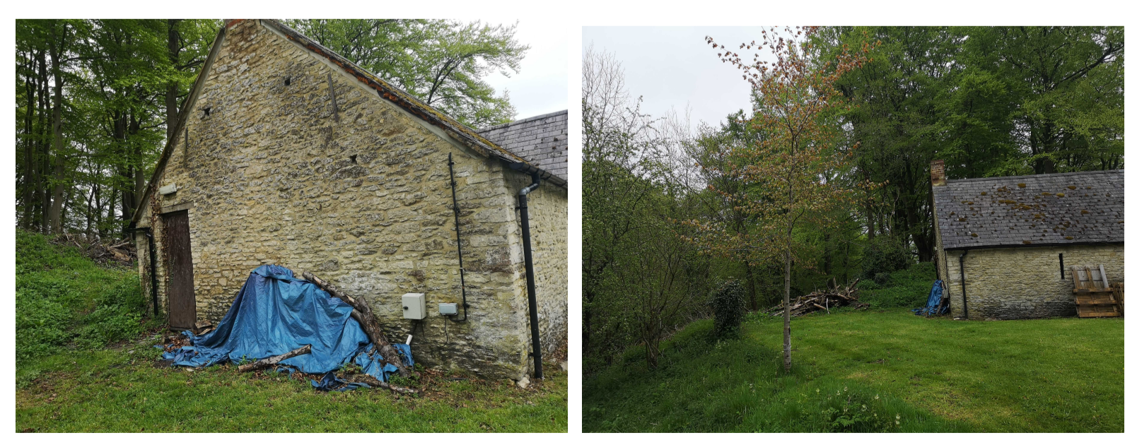
P/214 EXISTING STORE / PLANT SITE PHOTO
